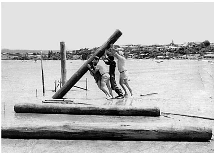
Placing the piles by hand.
